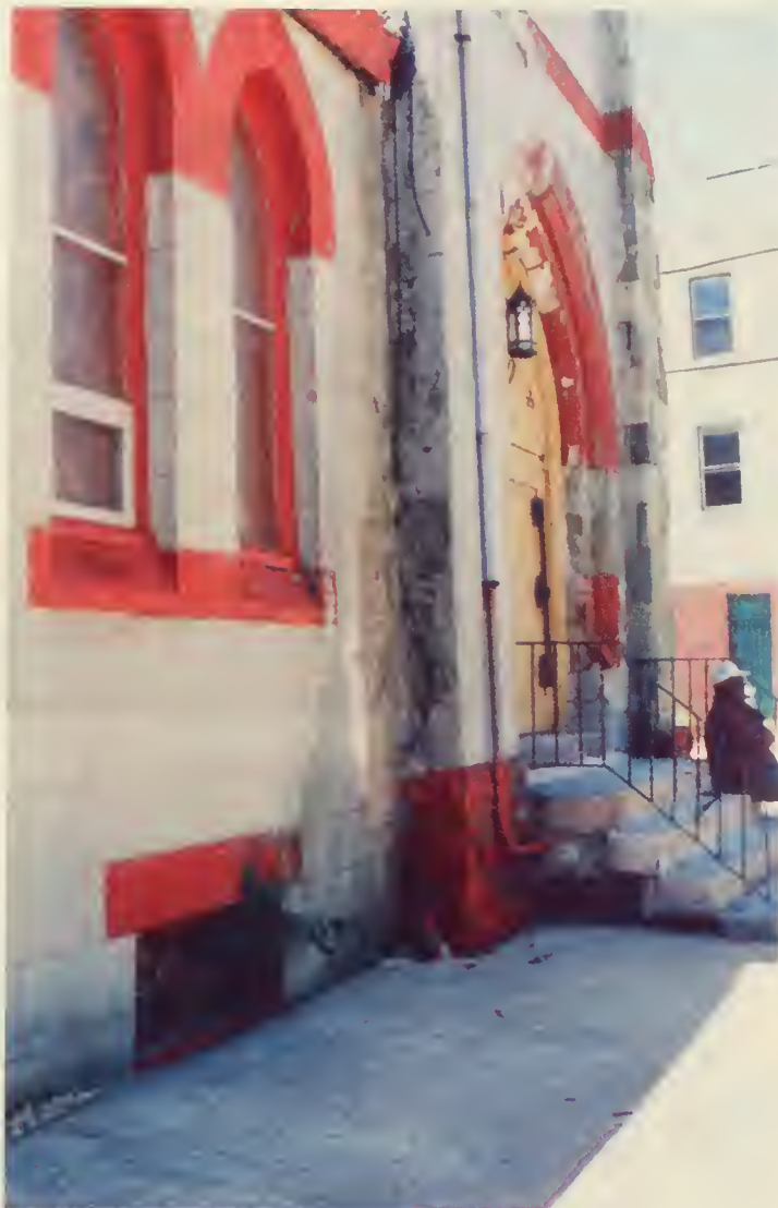
North Elevation of Church Building (K)
